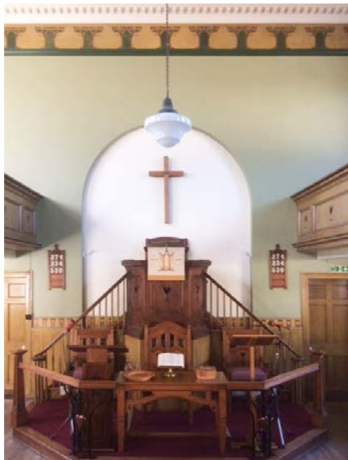
Completed restoration. Photo by Jackie Embury
