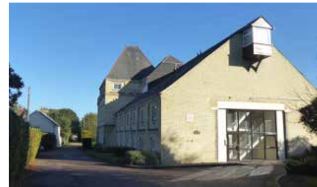
Figure 53: Former Fordham Maltings, Green Lane/Station Road
