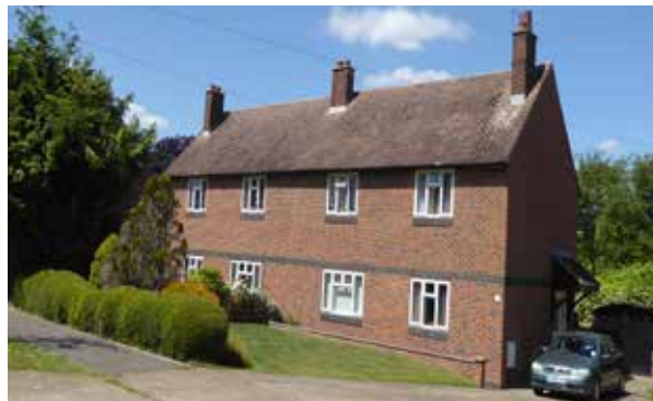
Figure 67: Brickwork with a decorative band
