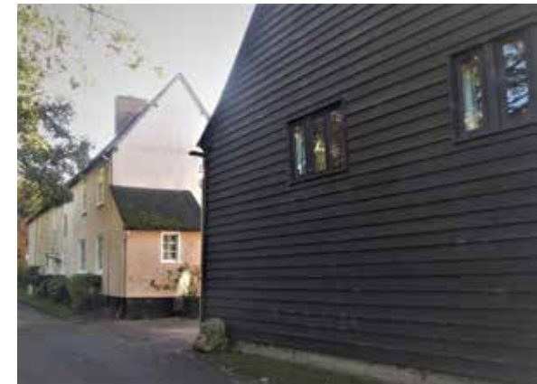
Figure 45: Example of weatherboarding, Ringstead Farm
