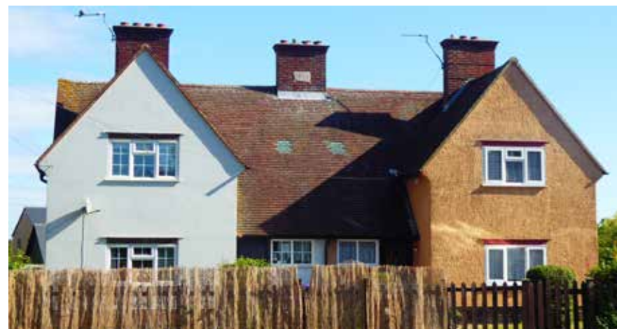
Figure 59: Example of 1920s housing 'fit for heroes', Station Road
