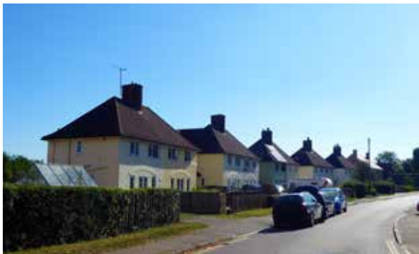
Figure 54: Station Road, looking north
